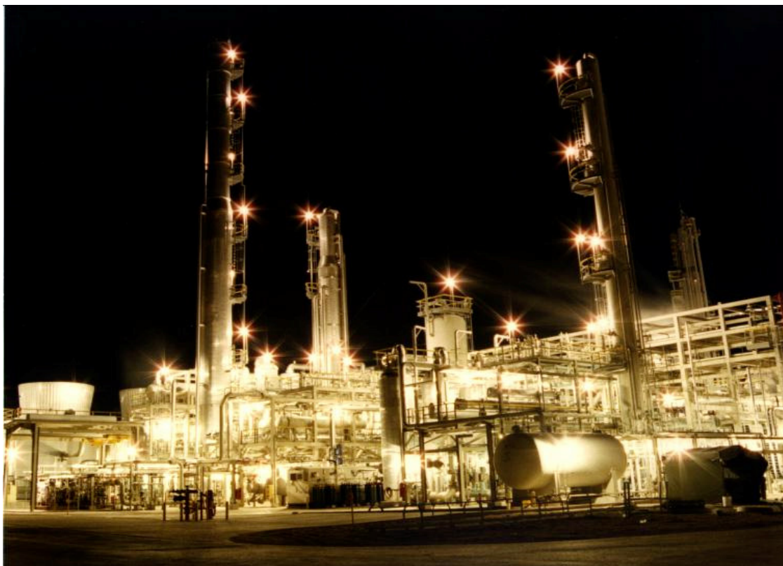
Photo: Modular Construction employed in an Ethylene Recovery Unit built by Pro-Quip for Mobil Chemical in Houston, Texas
